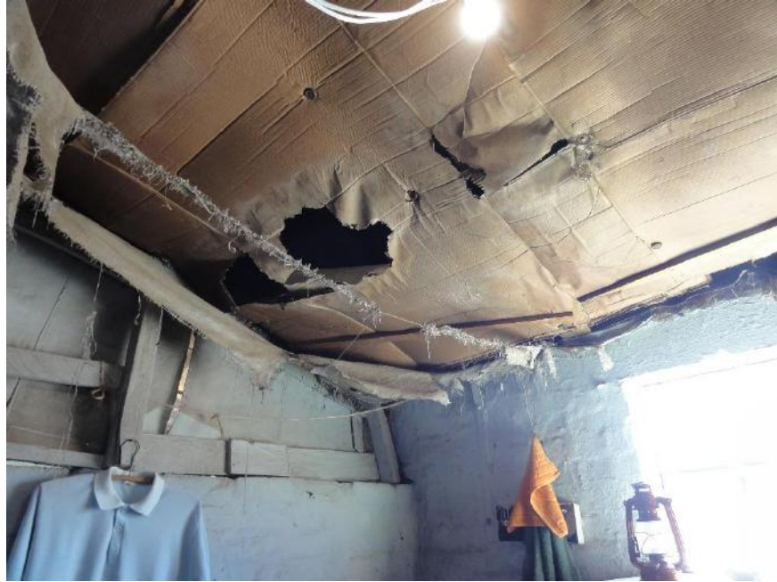
Fig 12. Sleeping quarters showing the use of cardboard for ceiling insulation and a paraffin lamp for light.
